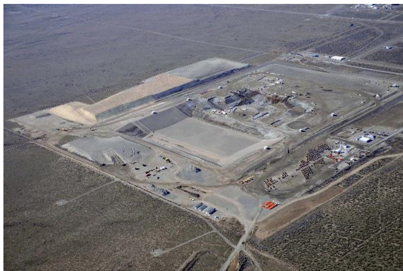
The Waste Treatment Plant under construction at Hanford.
