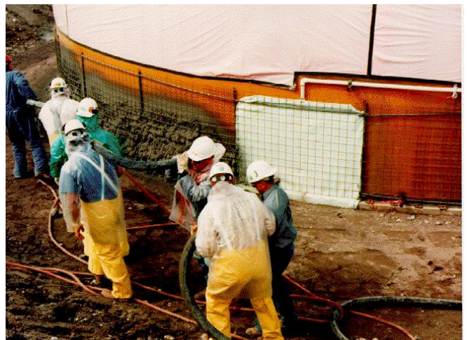
The Tank Farms: one of Hanford's most dangerous worksites.
