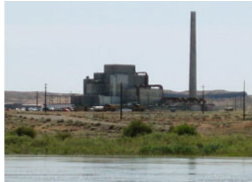
Birthplace of a bomb: This reactor building is part of the Hanford nuclear site in Washington state that produced the plutonium for the atomic bomb dropped on Nagasaki in 1945. KYODO PHOTO
